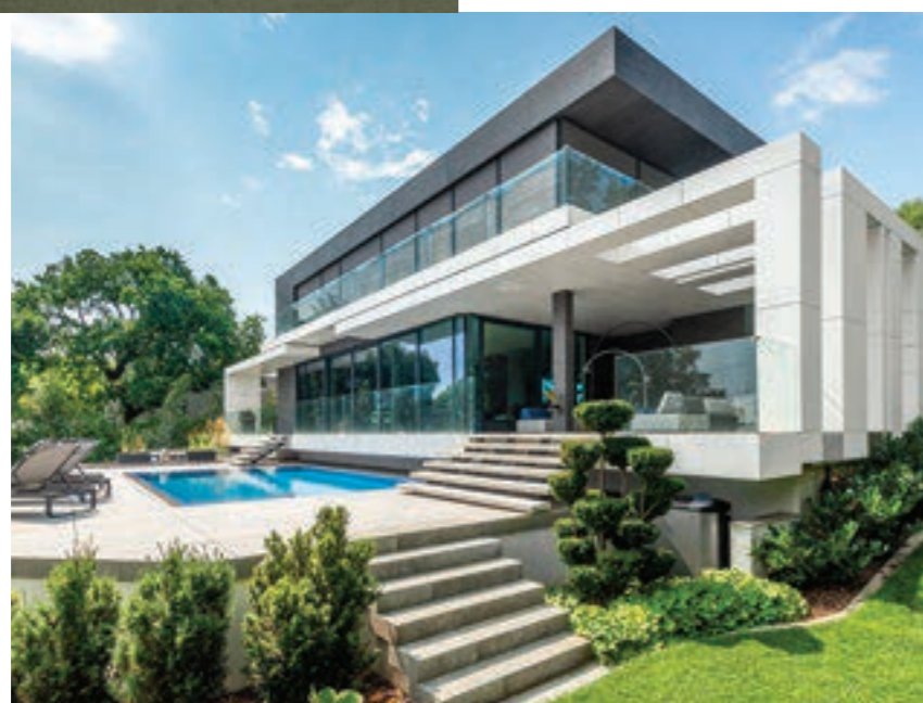
PRIVATE RESIDENCE - BENYEI ARCHITECTURE - BUDAPEST
